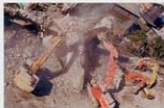
巨大なハサミで寸断される高速道路 Expressway structures being cut and removed using large scissors-like machines
