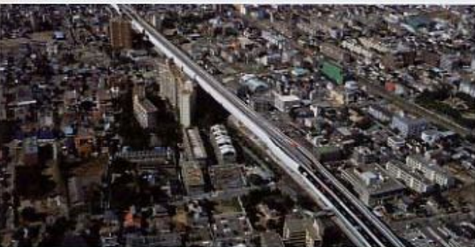
復旧後 Restored bridge
