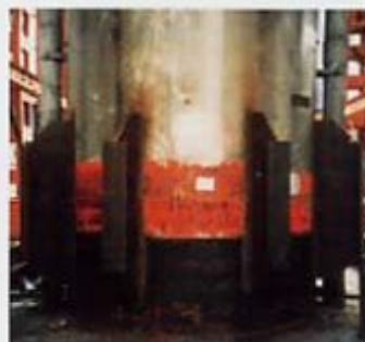
鋼製橋脚の2次災害防止のための応急補強 Emergency strengthening on a steel pier for secondary disaster prevention
