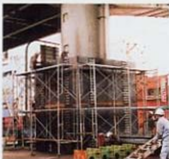
RC橋脚の2次災害防止のための応急補強 Emergency strengthening on a reinforced concrete pier for secondary disaster prevention
